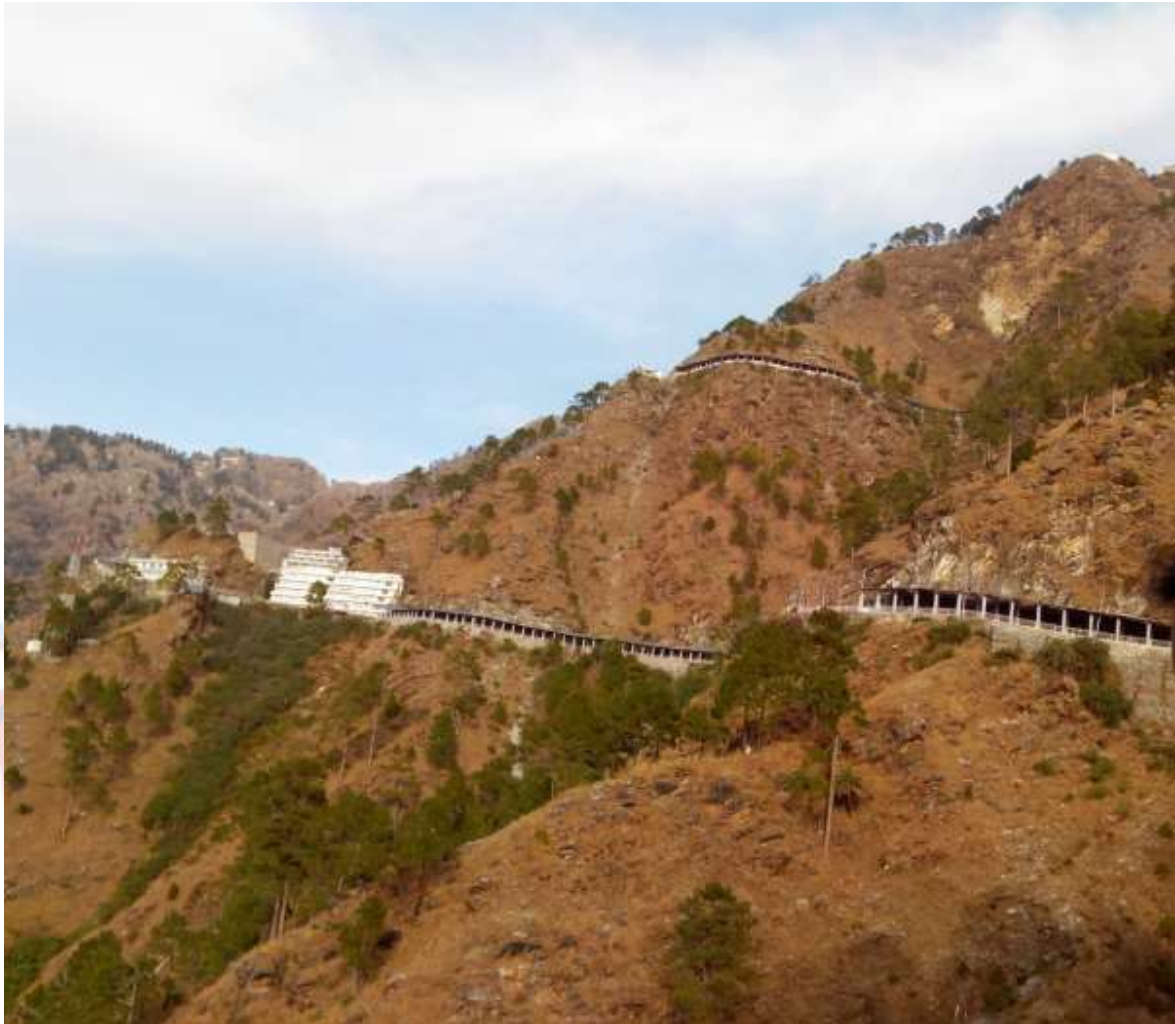
Figure 4: Landslide Prone Route of Vaishno Devi Shrine, Jammu and Kashmir
